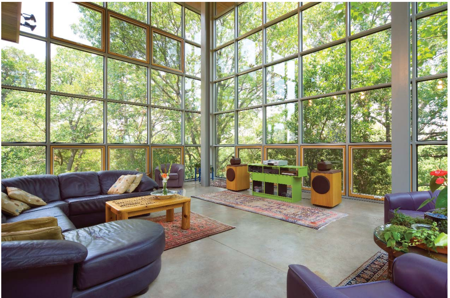
Offering the sensation of being inside a glass cube, the living room is eclectically furnished with an emphasis on the views. Supported by a grid of steel tubing, the windowed wall is 25 feet wide and 22 feet tall. Despite the height of the windows, the use of insulated, low-E glass and a geothermal HVAC system keep energy bills surprisingly low.
